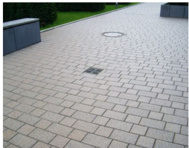
University building in Saarbrücken, Germany
